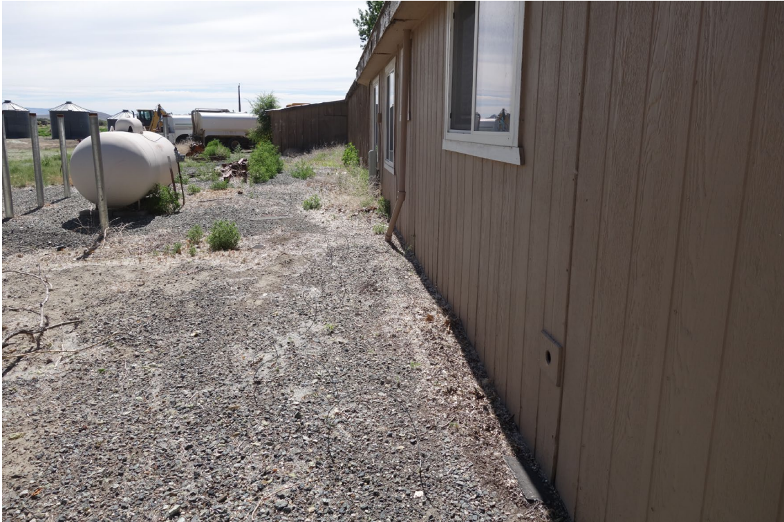
Mason Valley WMA Office / Headquarters - Building #0650 Description: View of Wood Siding Clearance to Grade.
