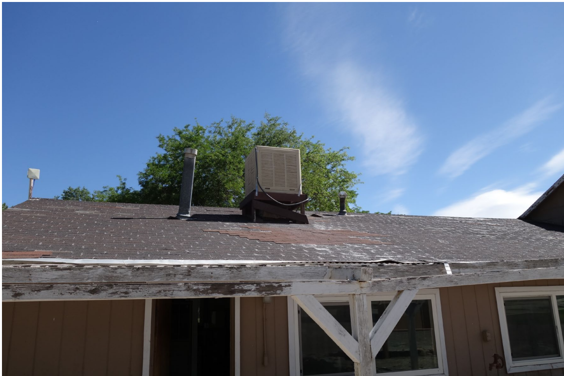
Mason Valley WMA Office / Headquarters - Building #0650 Description: Exterior of the Building & Roof Replacement Needed.
